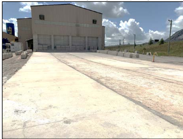
After Repairs – concrete was placed in strips.
