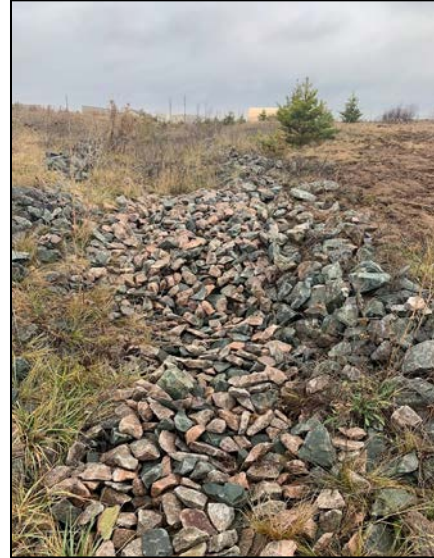
NCWIB #3 – After riprap repairs
