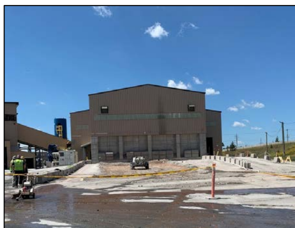
Before Repairs – old asphalt being removed.
