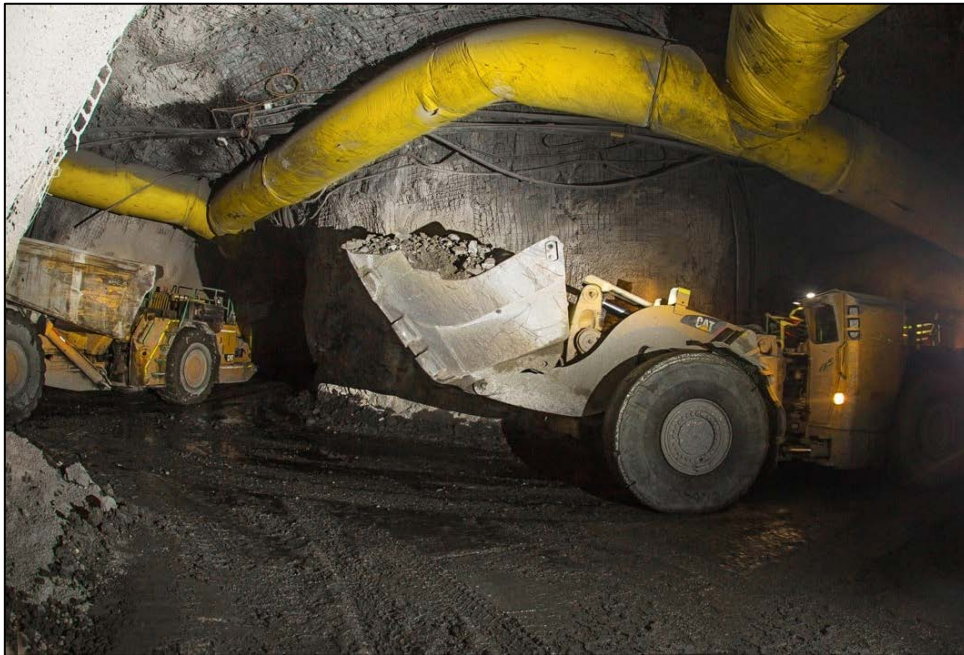
Haul truck loading material underground
