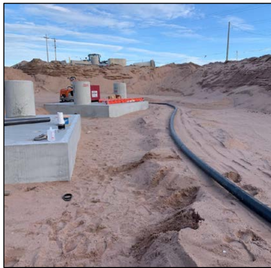
New connections between the tanks and forcemain
