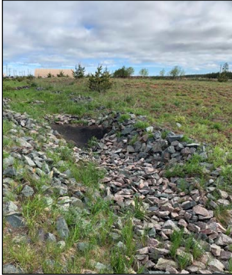
NCWIB #3 – Before riprap repairs
