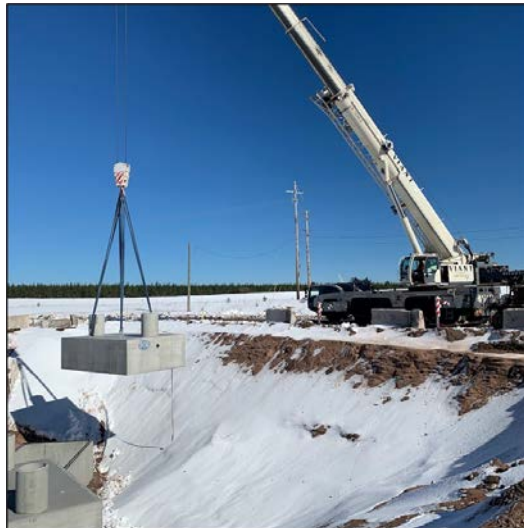
Placement of the top half of one tank
