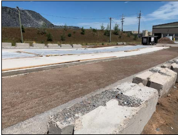
During Repairs – grading and repaving.
