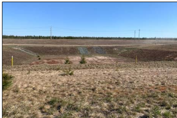
Non-Contact Water Infiltration Basin (NCWIB) #1 near the WTP
