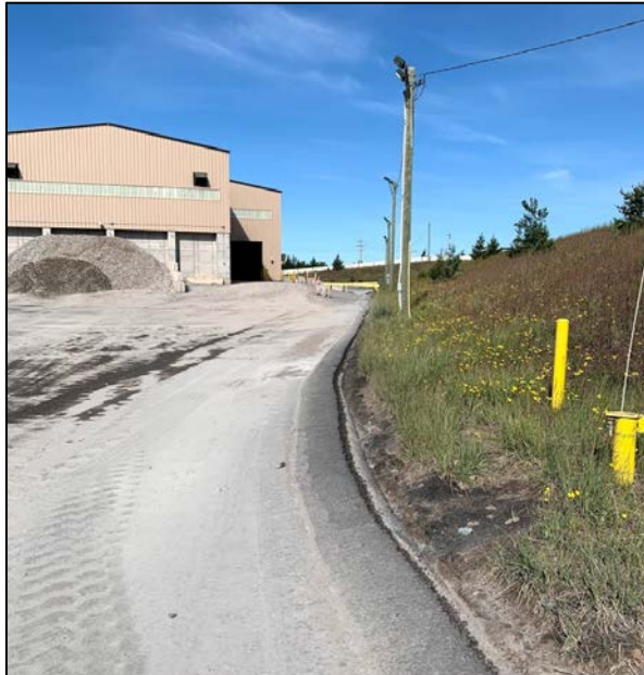
Curbing located near QAL067A
